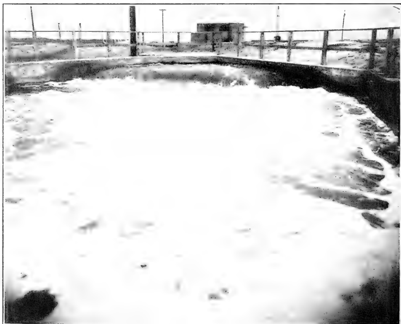
2. SEA WATER BEING PUMPED OVER DAM AT RATE OF 58,000 GALLONS PER MINUTE.
